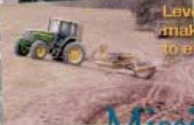
Levee Board crew and equipment make repairs to the levee slope due to erosions caused by rats
